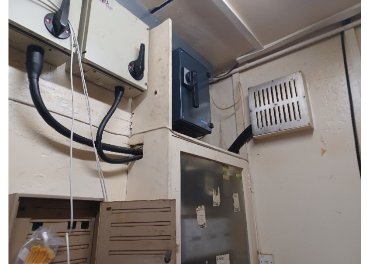
Photo showing existing electrical installation mains units and incoming supply
