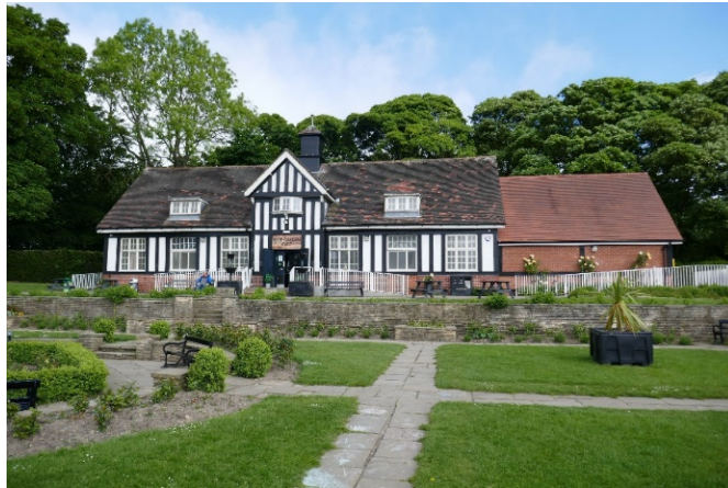
Photo of front elevation facing Rose Gardens
