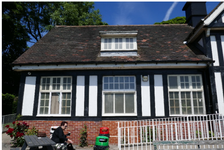
Photo of front elevation gable showing holes in the timber and render panelling, and the deterioration of the roof fascia, soffit and underside of window over main entrance.
